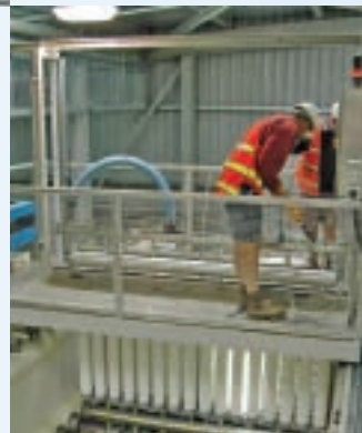
MemSAP™ (membrane service access platform) eases maintenance and repairs.
