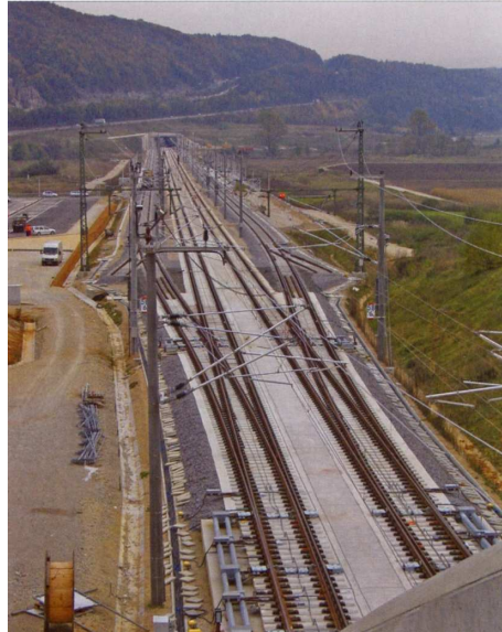
Mixed Use in Germany, an example: Nuremberg-Ingolstadt passing station for freight and high-speed trains.
